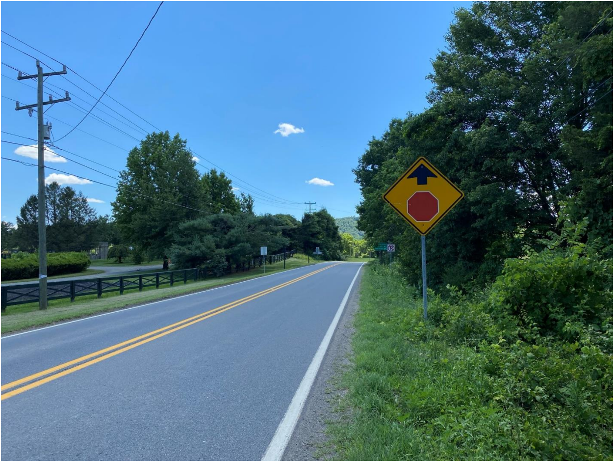
Figure A.4 Stop ahead warning for traffic approaching from Rte. 245
