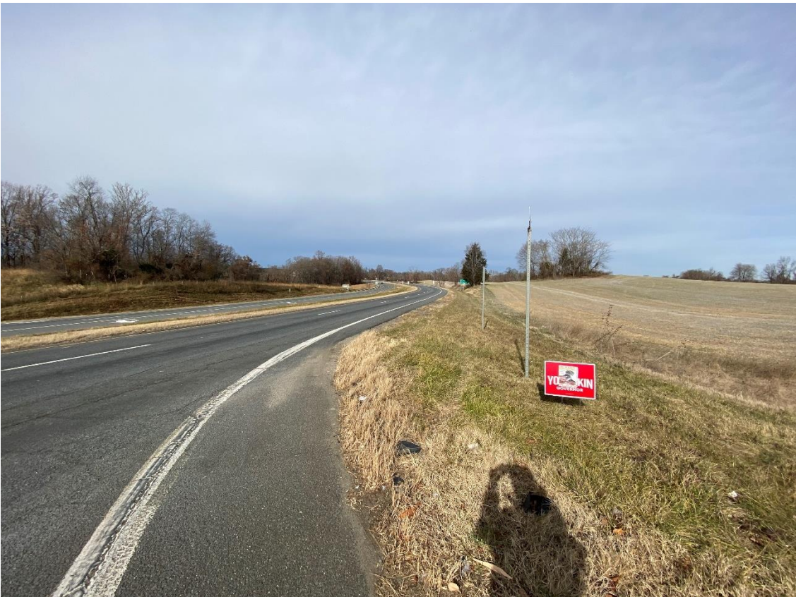
Figure 6: Looking North from Westbound Route 245
