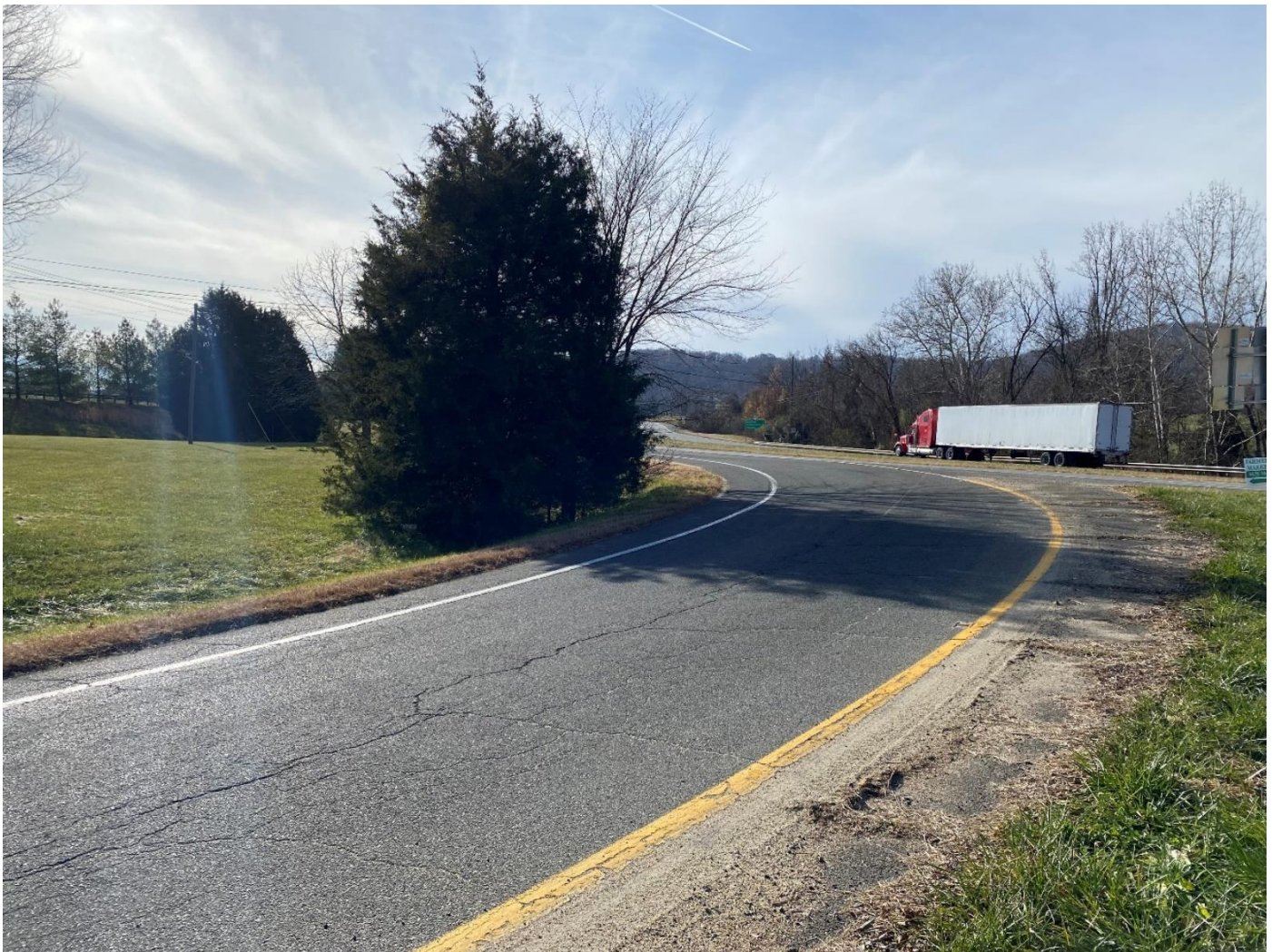
Figure 3: Tree Sight Obstruction on Westbound Route 245
