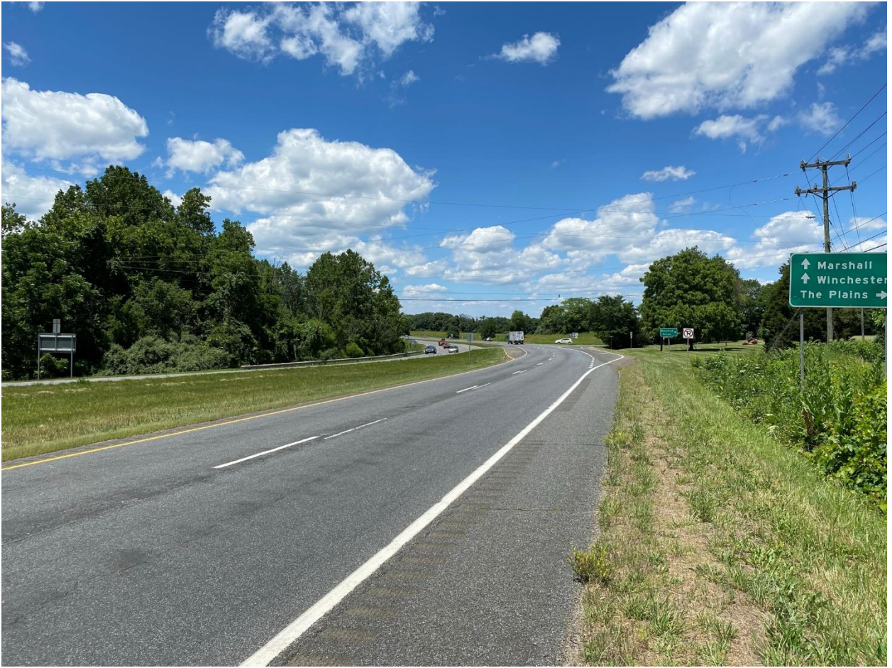
Figure A.8 View of intersection to traffic approaching from northbound on Rte. 17
