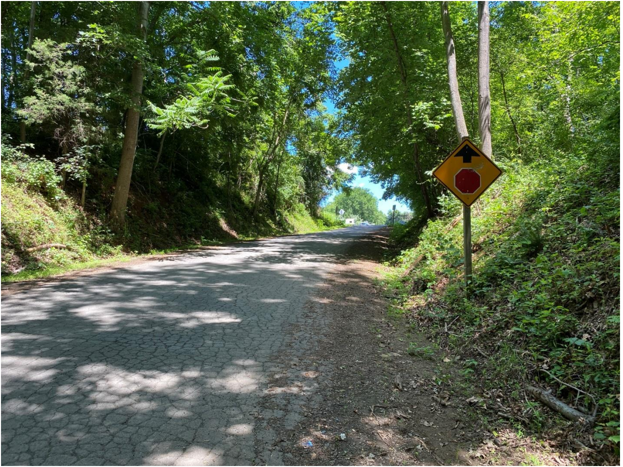
Figure A.7 Stop ahead warning for traffic approaching from Rte. 703
