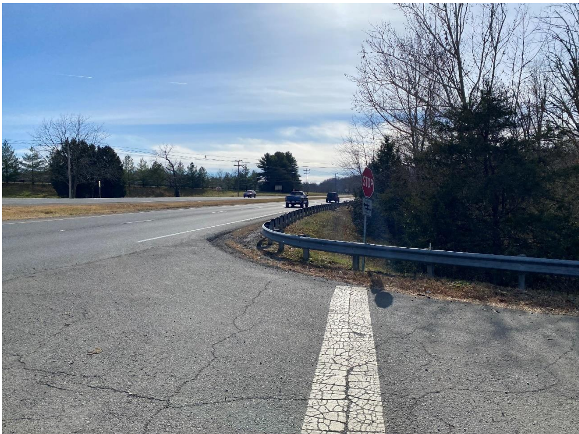
Figure 10: Looking South from Route 703 Eastbound
