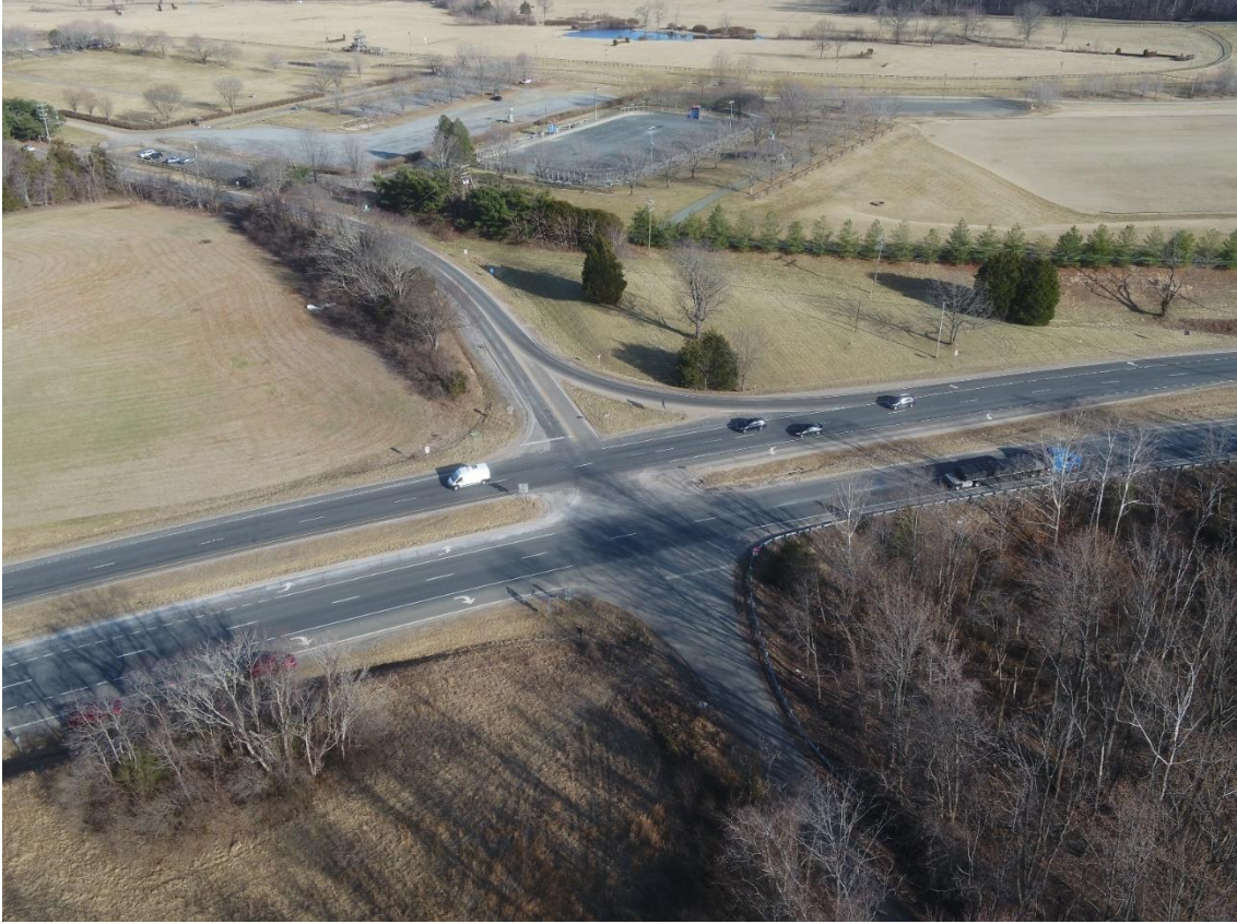
Figure 2: Route 245 Approach Aerial
