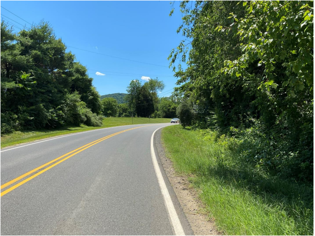
Figure A.3 Sight distance obstruction for traffic approaching from Rte. 245
