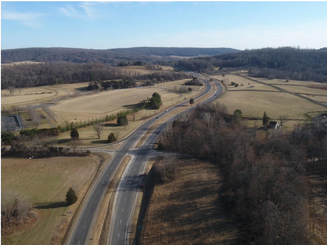
Figure 12: Aerial Image of US 17 South of the Intersection
