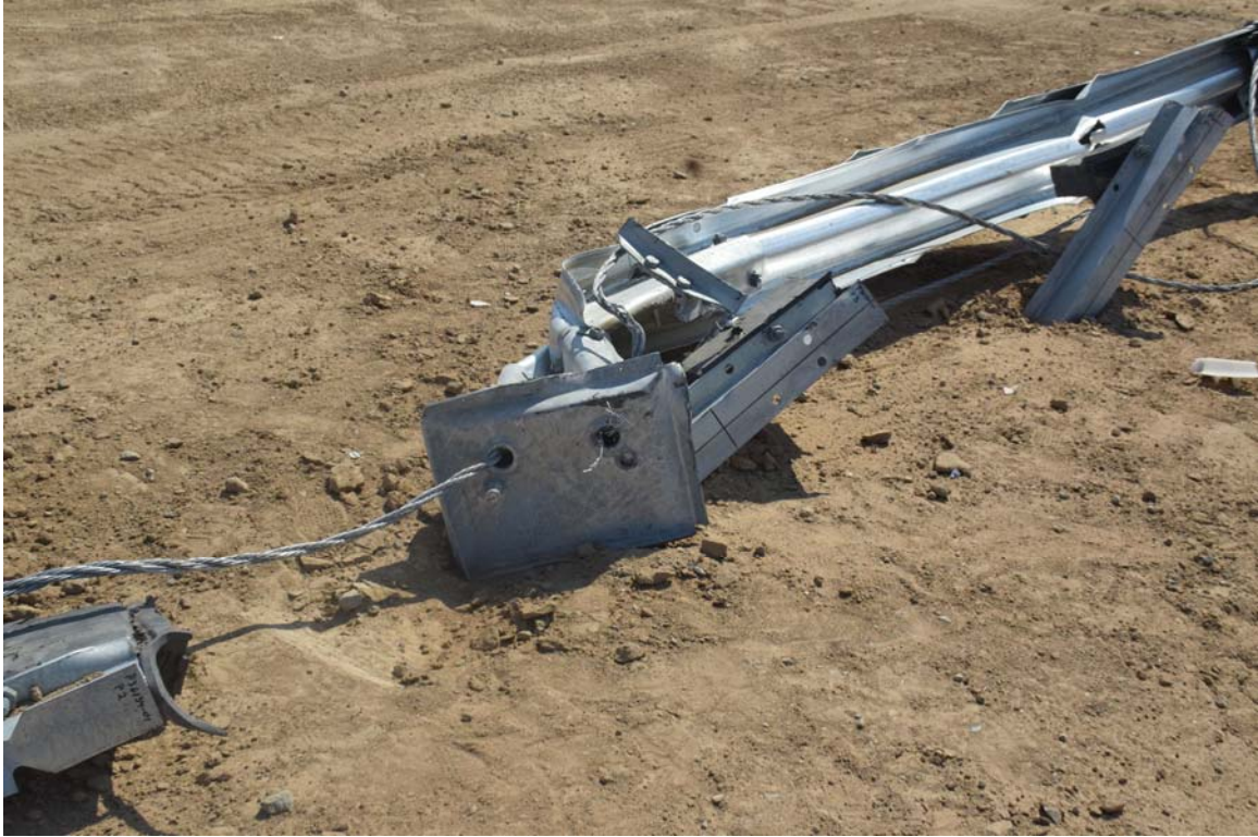
FIGURE 37. Test Article Damage
