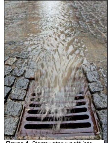
Figure 1. Stormwater runoff into drop inlet.
