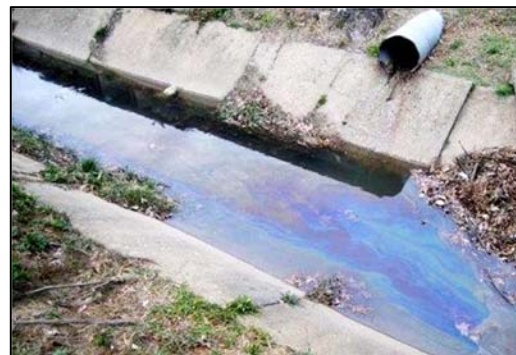
Figure 6. Illicit discharge of oil in a concrete stormwater conveyance ditch.
