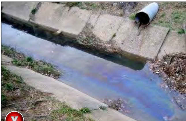
Oil sheen from illicit discharge in concrete-lined storm-water ditch.
