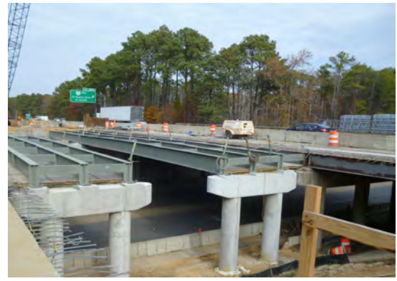
Figure 4.5.1.6 - Median Widened Bridge Construction
