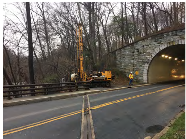
Figure 4.4.3.1 - Drilling in Close Proximity to existing NPS Bridge
