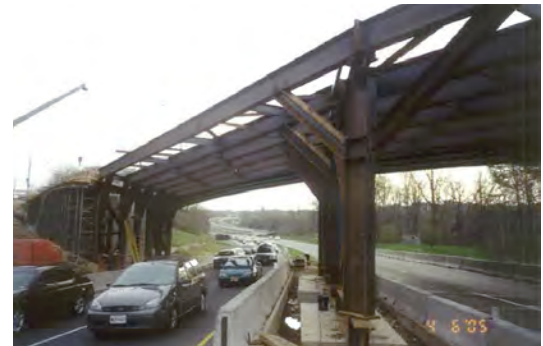
Figure 4.5.1.7 - Arch Falsework over Live Traffic
