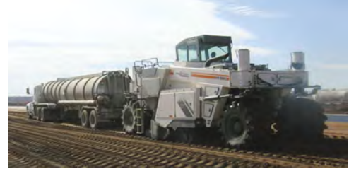
Figure 4.5.1.9 - Breaking Sled and FDR Process
