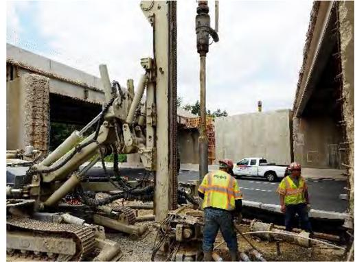
Wagman self-performs all non-disruptive foundations types (such as micro-pile pictured here on Route 7) controlling cost, schedule and reducing work zone requirements.
