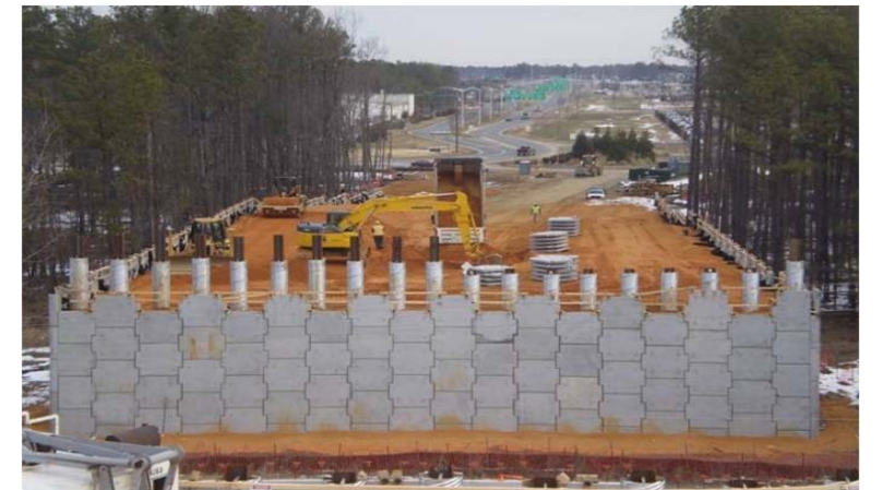
MSE Wall Construction for a Bridge Approach
