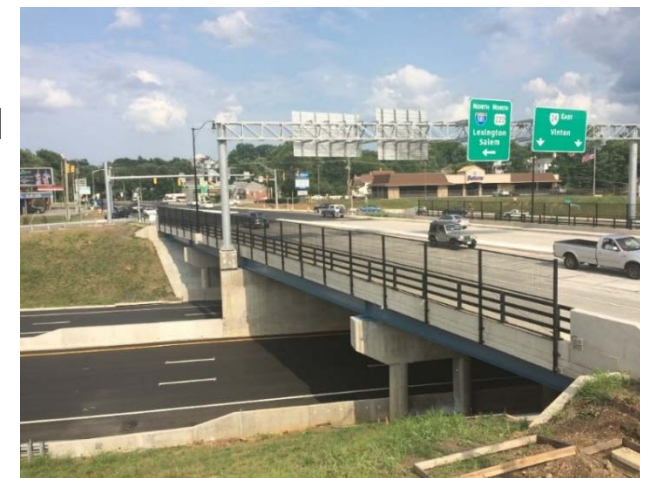
Post Construction I-581 at Elm Avenue Interchange
