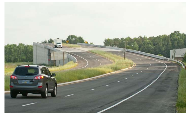
Post-Construction on Airport Connector Road
