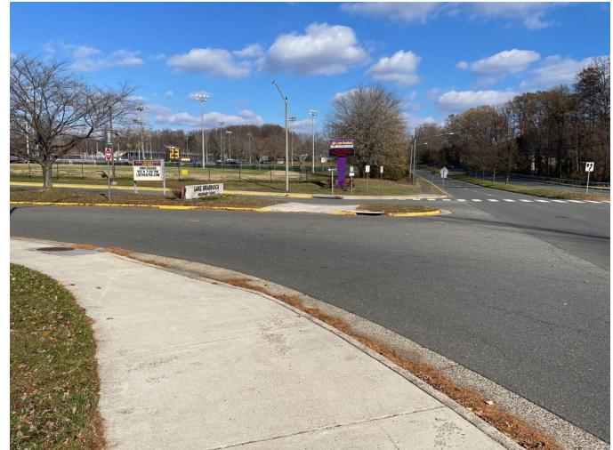
Figure 23: The crosswalk across the school main access driveway is unmarked.
