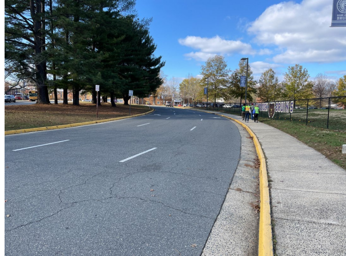
Figure 15: There are concerns about motor vehicle speeds on the school's main access driveway.
