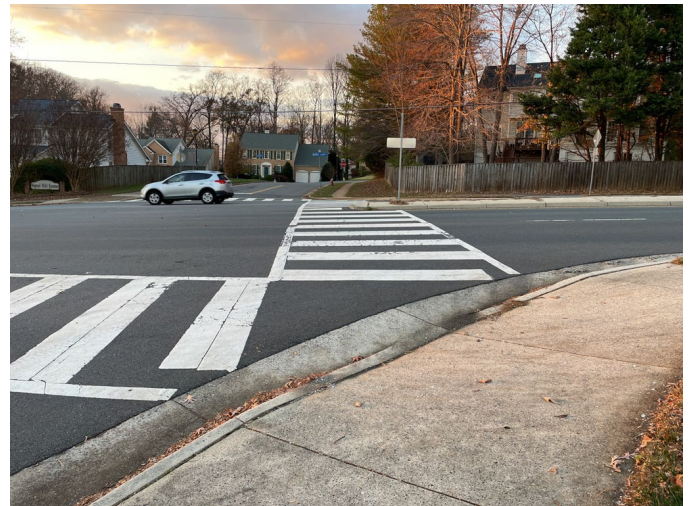
Figure 24: Uncontrolled crosswalk across Burke Lake Road at Signal Hill Drive.
