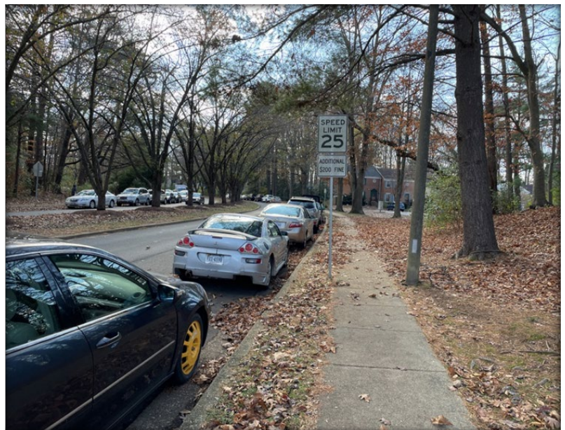
Figure 25: Sidewalk on Lake Braddock Drive
