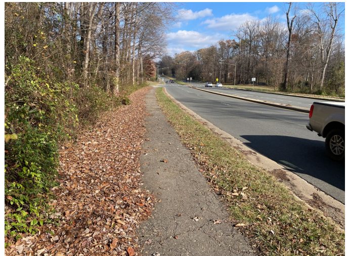
Figure 16: The shared use path on Burke Lake Road is approximately 6' wide.
