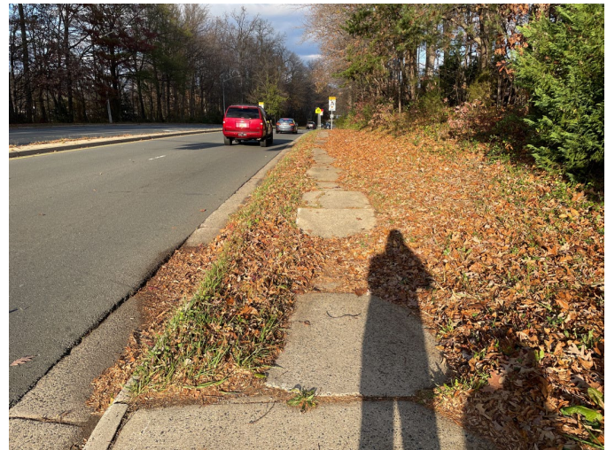
Figure 17: The sidewalk on the south side of Burke Lake Road is obstructed by leaves. There are also vertical discontinuities in the sidewalk that make it inaccessible.
