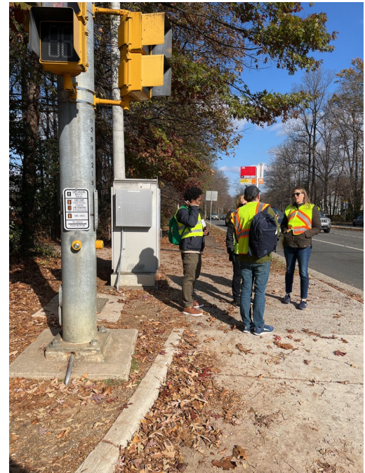
Figure 18: Pedestrian pushbutton is not accessible to people who use wheelchairs.
