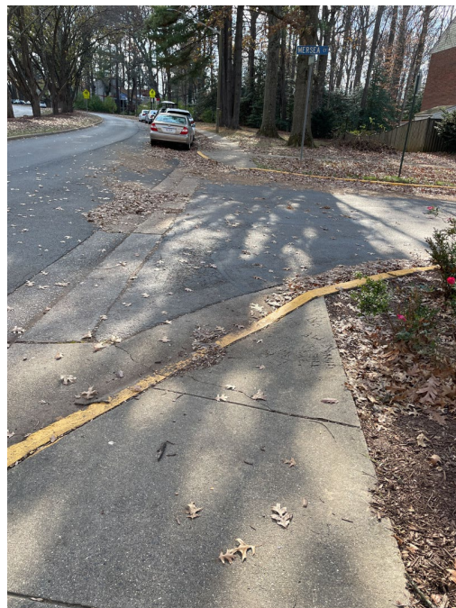
Figure 27: Crosswalk across Mersea Court (south side) at Lake Braddock Drive.
